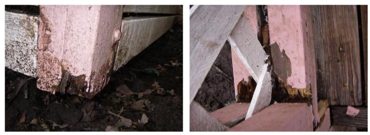
There is section of fascia above the front door that is in contact with the roof and has moisture damage. We recommend that the damaged fascia be cut away. It appears that the damaged area can be removed and no additional material be installed.
